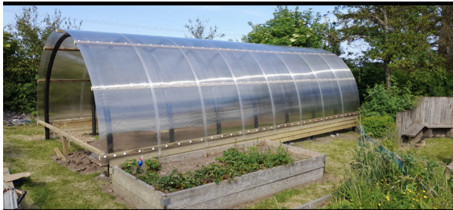
New sturdy polytunnel in an exposed sea-side location (Bracoden Primary School)
